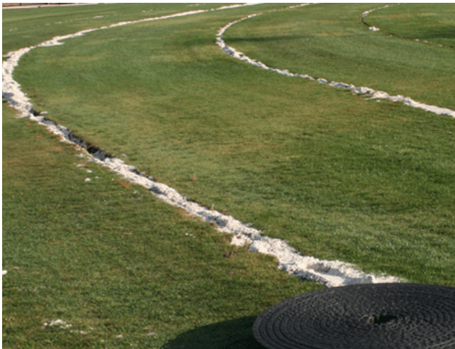
Underdrains being installed in the outfield of a softball field. Photo: Hydraway
