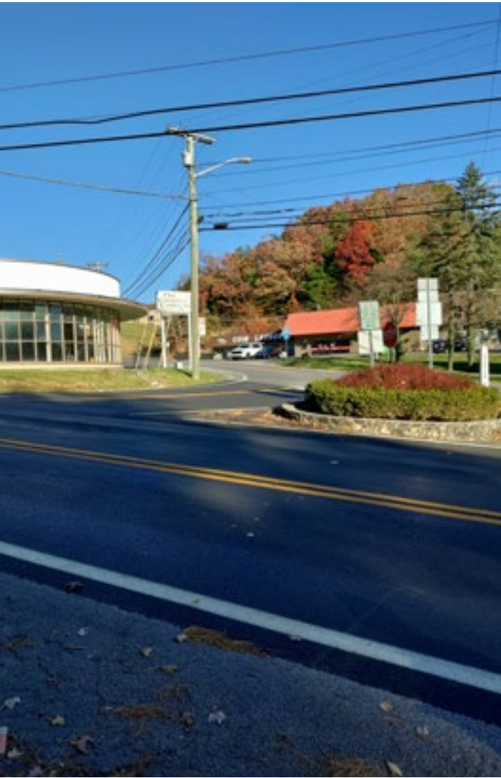
Sight distance is limited at the intersection of Stadium and Cherry Drive due to horizontal and vertical curvature
