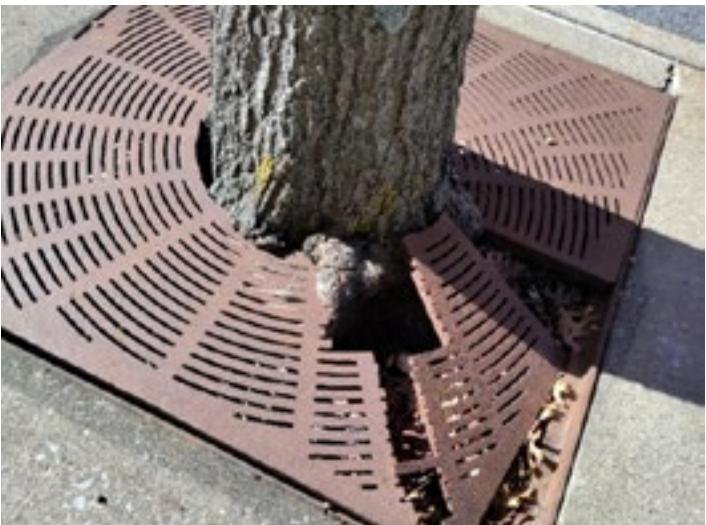
Photograph 24 Overgrown tree roots damage sidewalk and root cage
