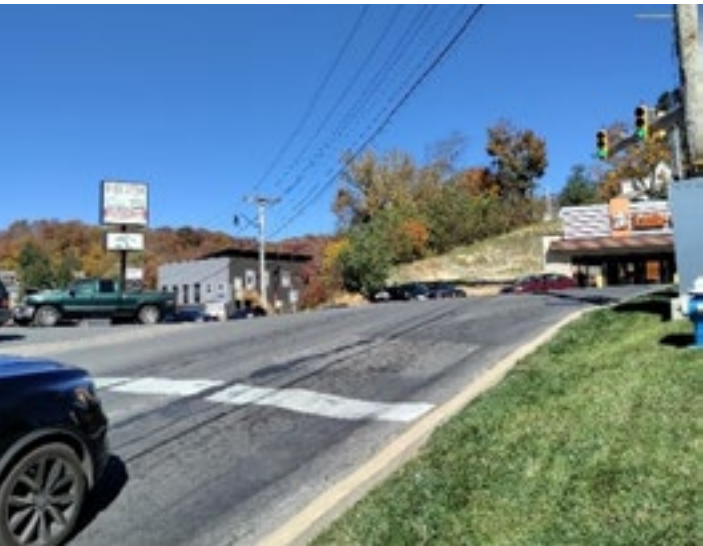
Photograph 29 Sight distance issues travelling east along College Avenue towards Bland Street difficulty seeing traffic from stop bar due to vertical curvature
