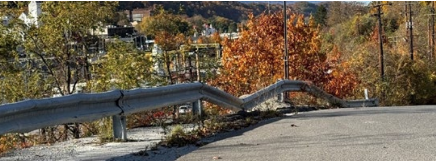
Photograph 50 Damaged barriers along Hardy Street to Orange Street
